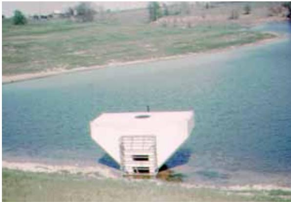
*A concrete tower connected to a pipe extending through the dam serves as a principal spillway for most dams, controlling the water level. A slide gate at the bottom can be opened to lower the water level even more to allow maintenance or repair.*
