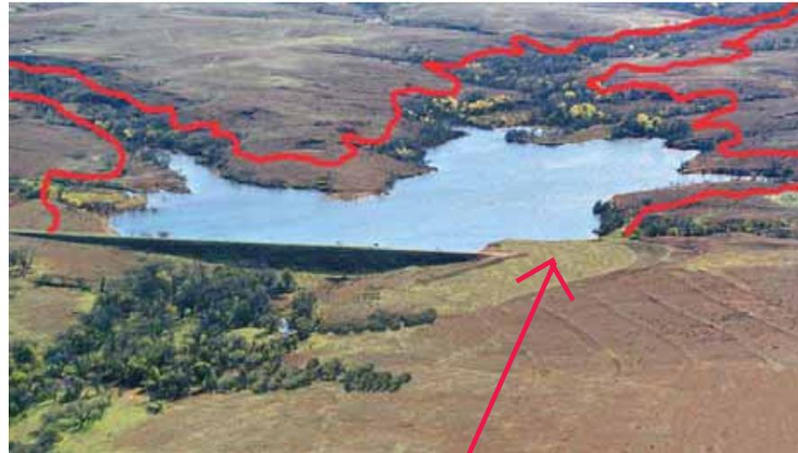
*When there is more water than the lake can store and the principal spillway can release, water will flow through the auxiliary spillway.*
