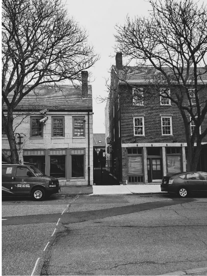
Photo 5, North Elevation, April 2024
