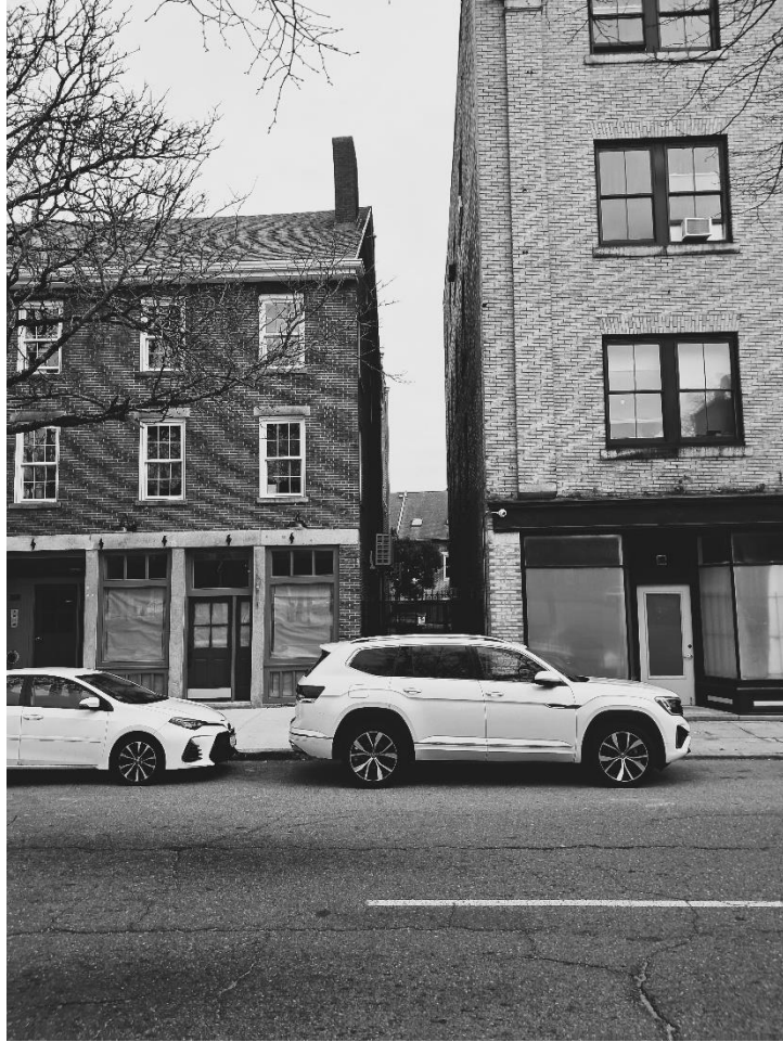
Photo 6, South Elevation, April 2024
