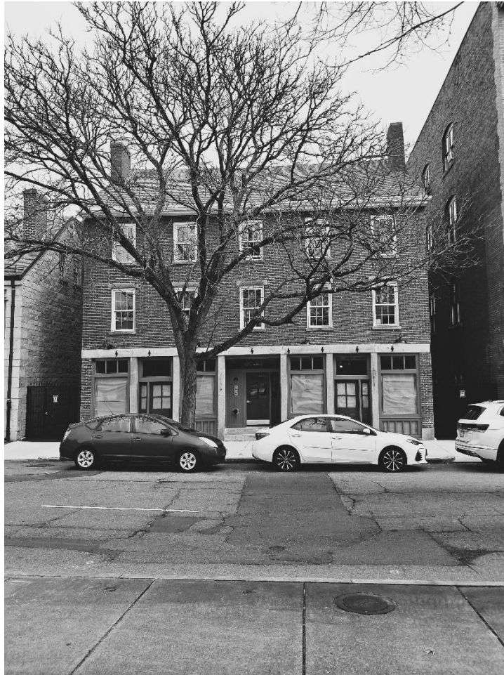
Photo 1, West Elevation, April 2024
