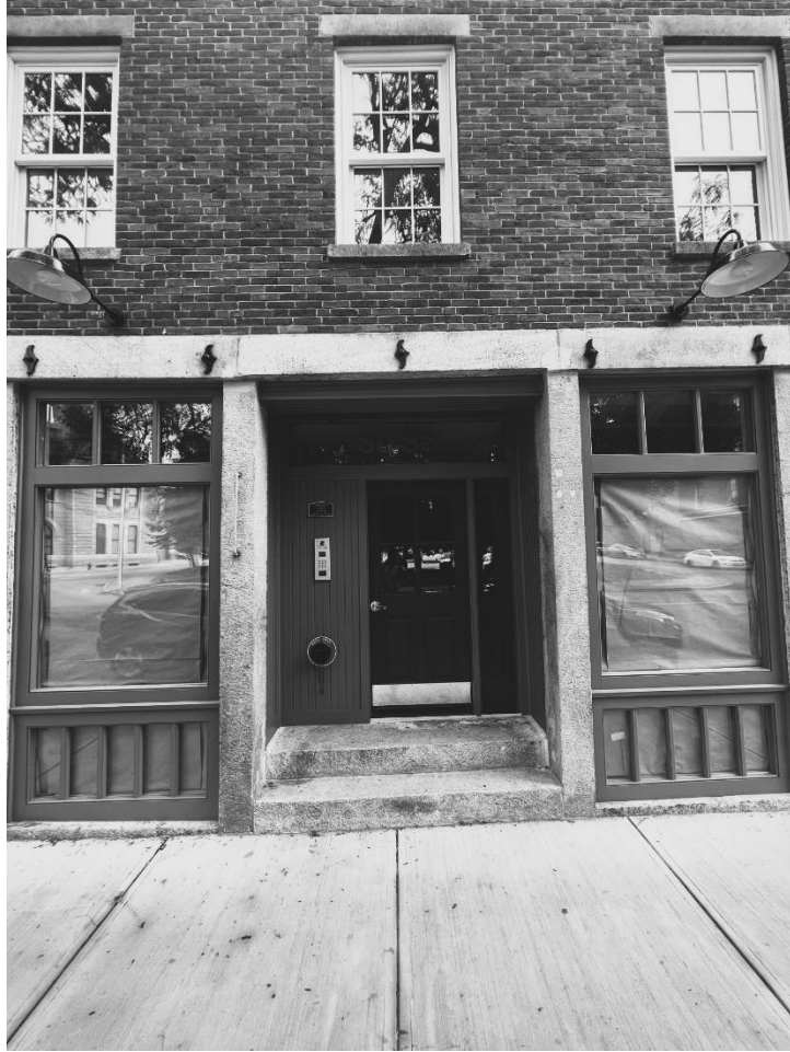
Photo 2, West Elevation, September 2023
