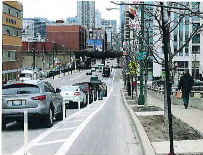
Shifted parking lanes and painted buffer zones (as space allows)-thermoplastic single lines \$0.40/LF; symbols \$4 each; painted lines \$0.04/LF
