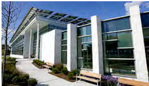
The North Shore Community College has just opened a Health Professions & Student Services building that is the first state ZNEB (Zero Net Energy Building) and LEED gold. It uses a combination of ventilation, lighting, a green roof, building orientation, chilled beams, geothermal energy, and photovoltaics.
