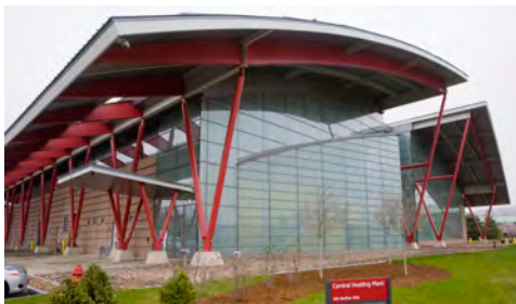
U Mass Amherst Cogeneration Plant
