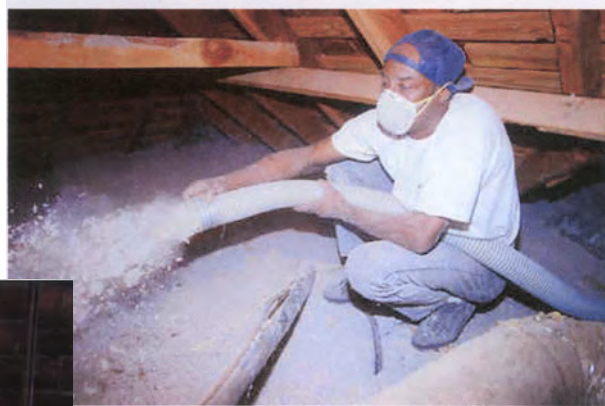
Cellulose loosefill insulation being blown into attic tasconindustries.com
