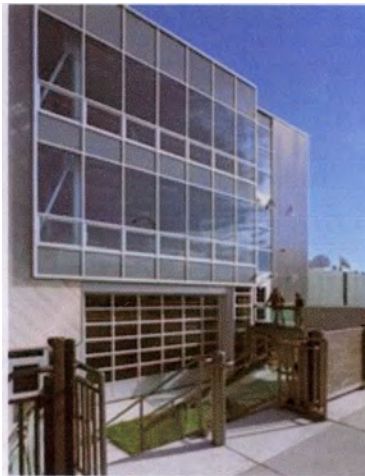
Artists for Humanity Arrowstreet, Architect
