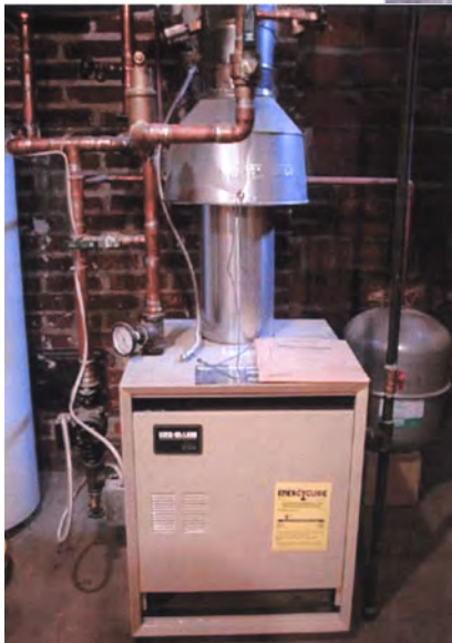
Energy efficient boiler
