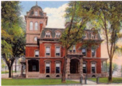
N Adams Public Library with 12kW of PVs & a geothermal heat pump
