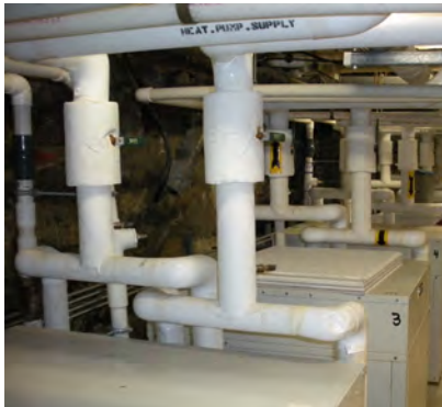
The 1.3 million sq.foot. Monarch Mill in Lawrence is heated & cooled with 60 geothermal 150 foot deep shafts Geothermal pumps in Quilt Museum
