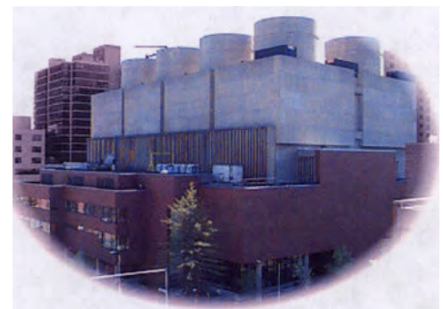
Medical Area Total Energy Plant located in the Longwood Medical Area serves steam, chilled water, and electricity to 9 million sq feet of LMA facilities.
