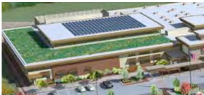
*The Hannaford Supermarket in Augusta, Maine became the first LEED certified supermarket with geothermal wells, PVs, a green roof, insulated skylights, & solar tubes for natural light, sliding insulated glass on freezers, low flow fixtures, etc. It was constructed in an abandoned high school.*
