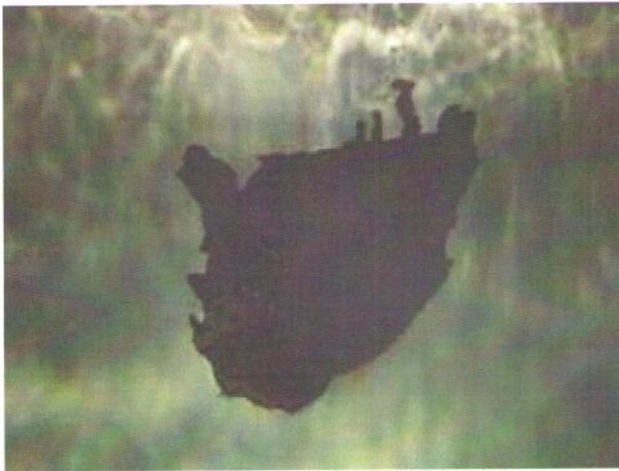
51 Interior Wall With Coating Loss, Exposed Underlying Steel, Mild Surface Corrosion And Mild To Moderate Staining
