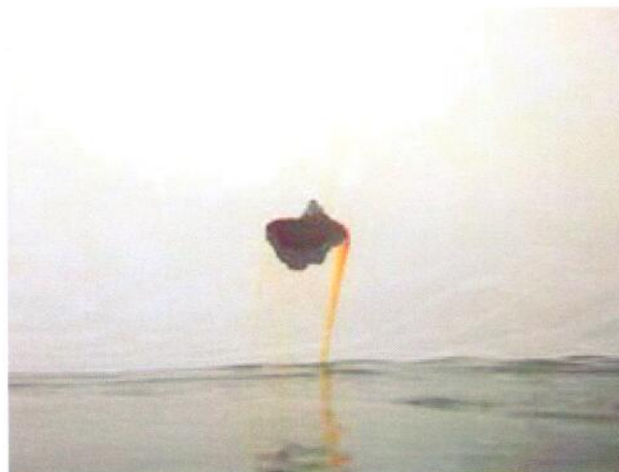
53 Interior Wall With Coating Loss, Exposed Underlying Steel, Mild Surface Corrosion And Mild To Moderate Staining
